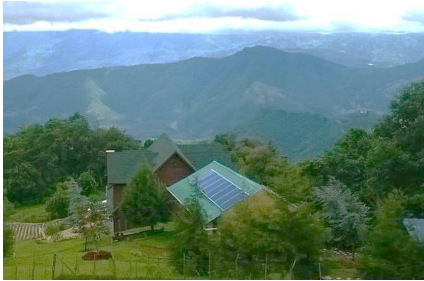
Figure 7. Photograph of a photovoltaic device installed in a Guatemalan's house
