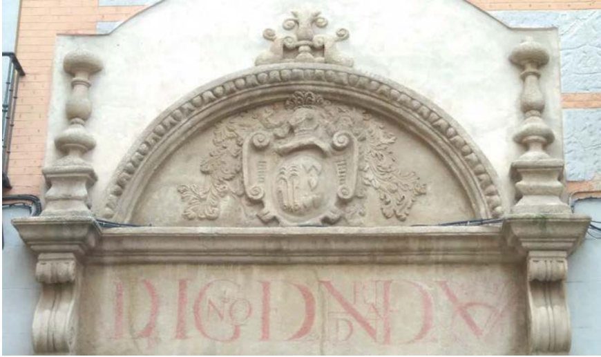
FIGURE 1 Frontage of the de la Palma family home in Toledo SOURCE: AUTHOR'S PHOTOGRAPH
